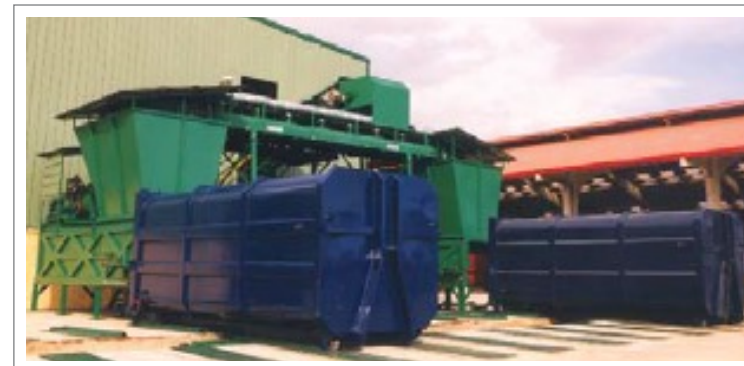
Partial view of the transfer station: compactor situations for multi-lifting equipped trailers
