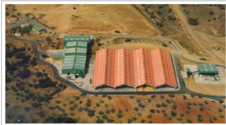
Aerial view of the waste treatment and transfer plant of the commonwealth of "La Vega" in Seville (SPAIN)
