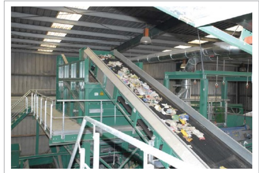
Conveyor belt with waste classification
